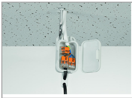
Pendant light connection in suspended ceilings
