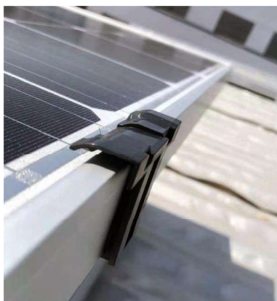
Figure 5 Drainage clips was installed
