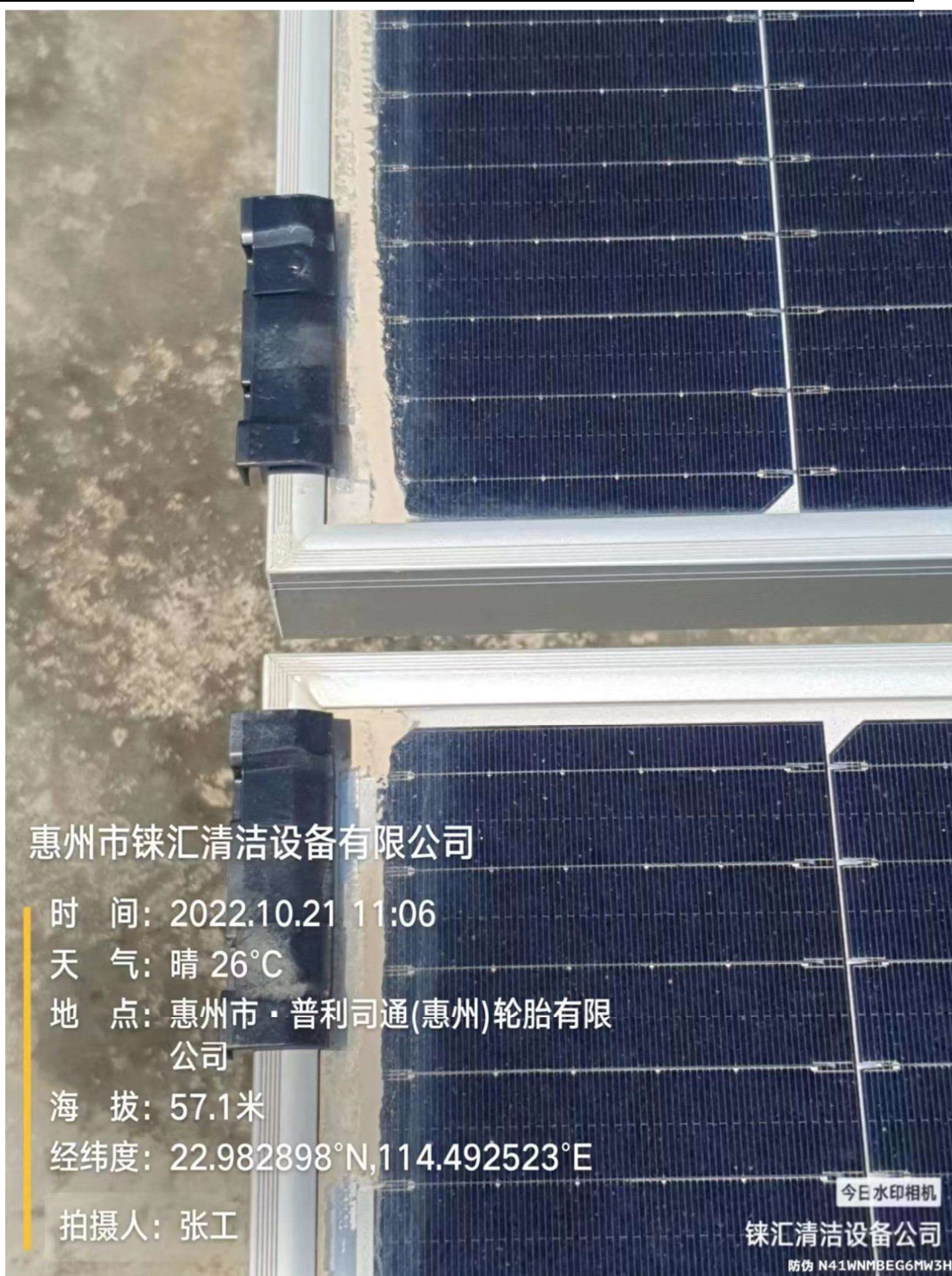
Figure 31 Soiling bands after light rain stops
