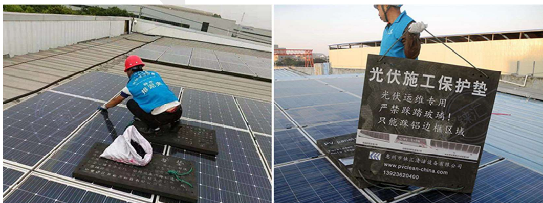
Figure 30 Installing drainage clips using protection mat
