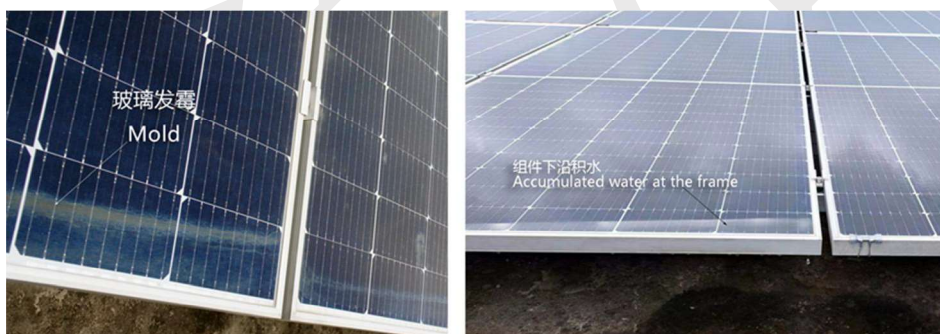
Figure 2 Moldy along the lower edge of the panels and accumulated water at the frame
